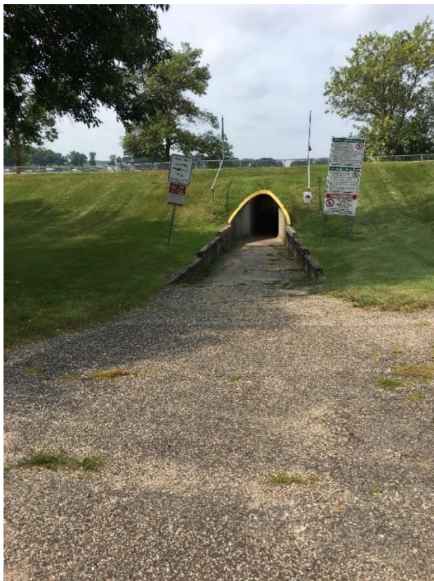
Figure 4. Cattle Pass Culvert
